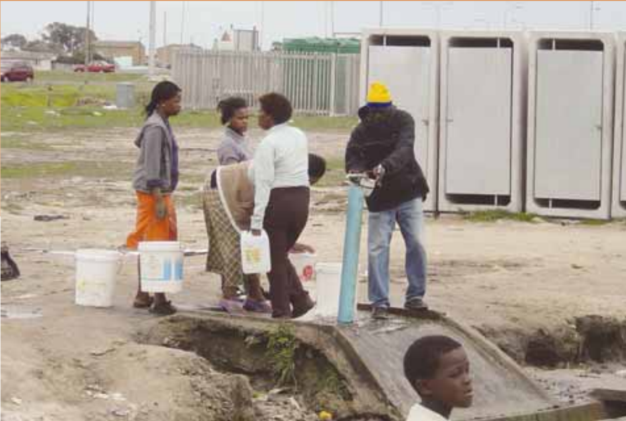
Communal water standpipe in Joe Slovo informal settlement outside Cape Town. Such standpipes represent the basic level of water service the government of South Africa wishes to guarantee to all citizens. Photo credit: Anton Earle.
