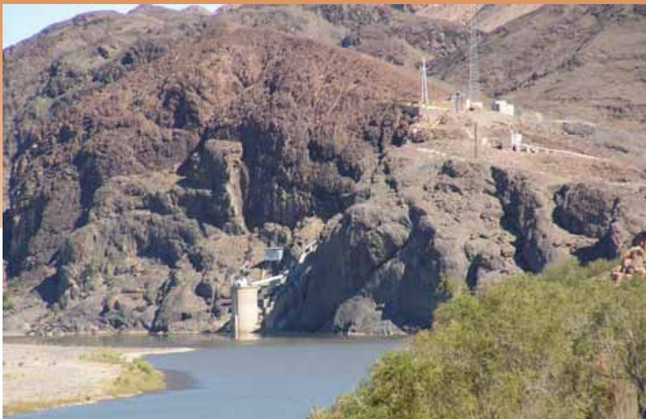
Pumping station pumping water from the lower Orange River to the Namibian mining town of Rosh Pinah. Photo credit: Daniel Malzbender.
